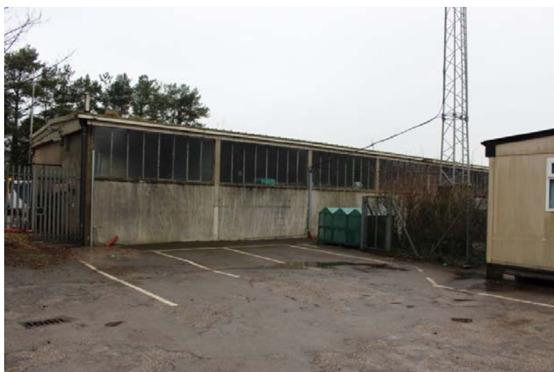
Photo 28 Prefabricated buildings site 88
